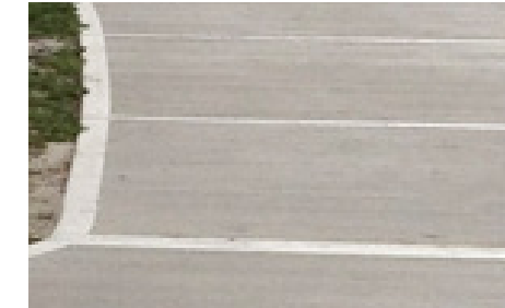
Brushed Concrete with trowel edge finish (streets)
