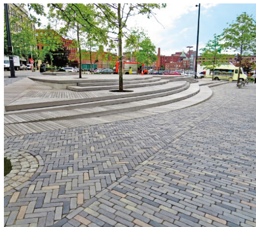
Paving to Street
