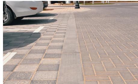
Flush Slipform Concrete Kerb
