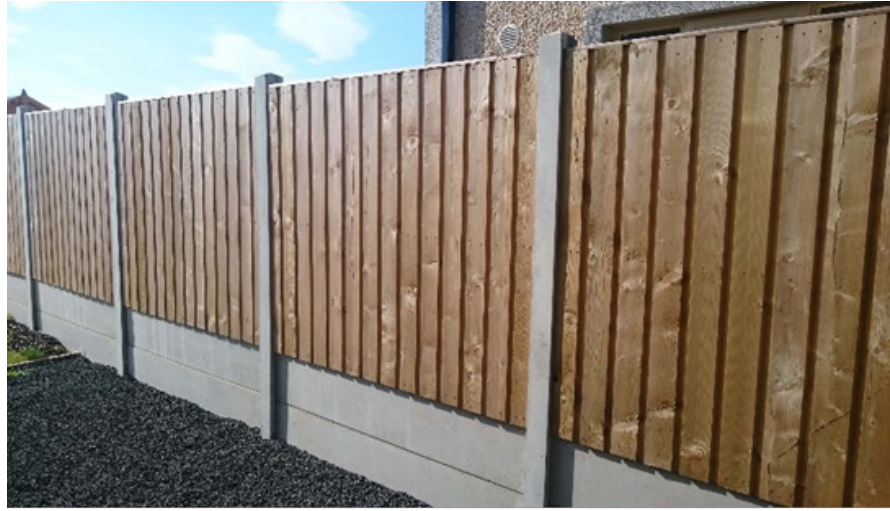
Concrete Post & Wooden Panel Fence
